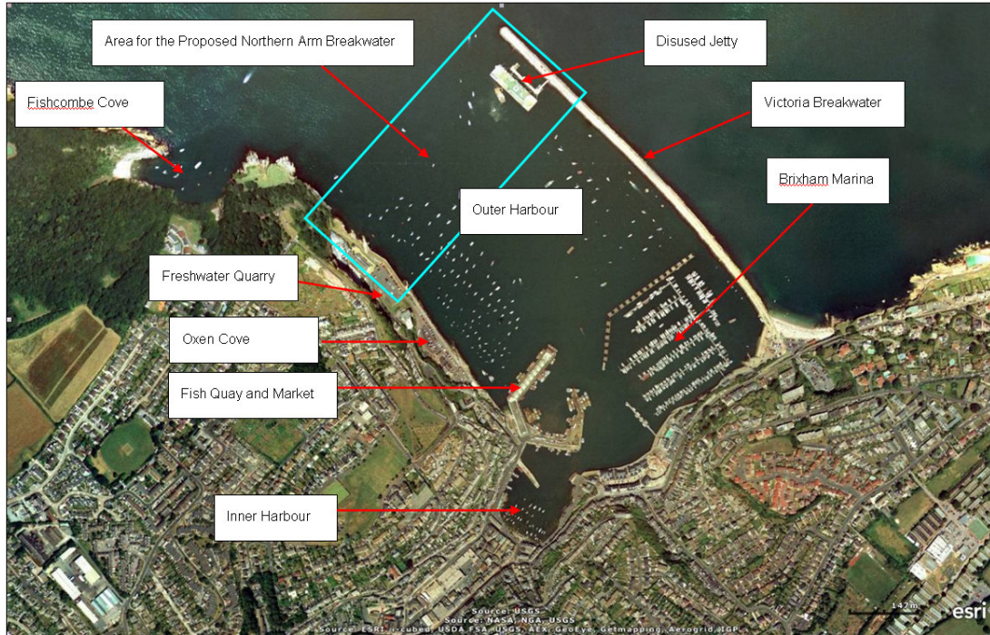
Figure 1.1 Aerial Photo of Brixham Harbour showing the Location of the Northern Arm Breakwater
